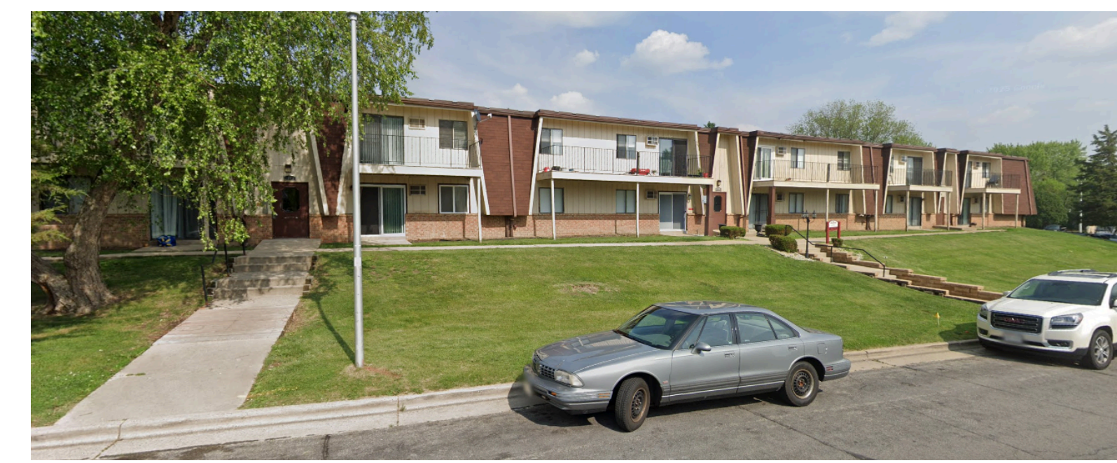
2A/A000 EXISTING - ALONG RED ARROW TRAIL 2
