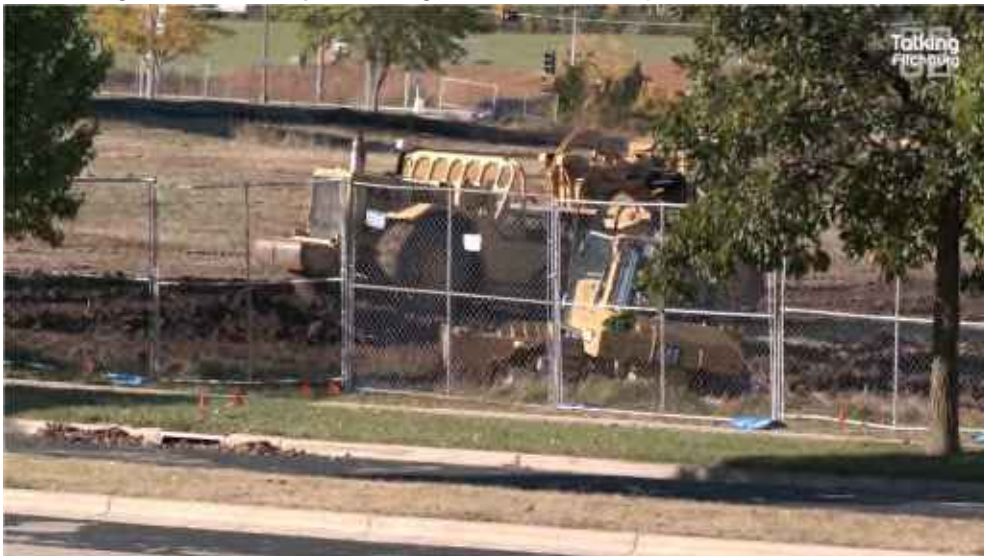
Fitchburg Public Safety Building Construction Update.
