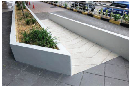
The ADA ramp is incorporated in the stair entrance and meets the needs of all users.
