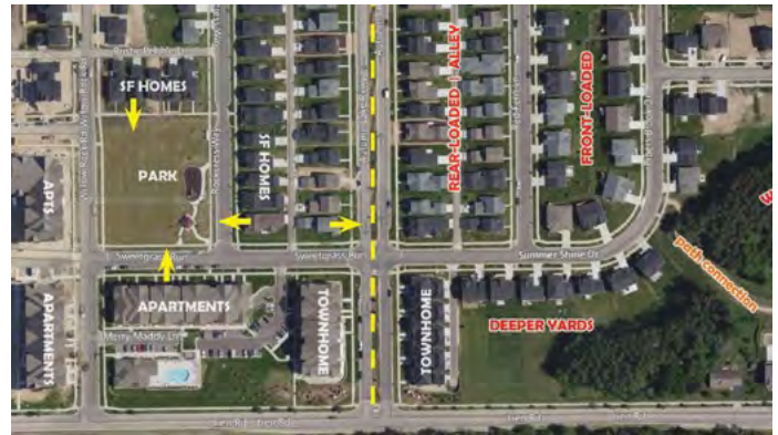
This neighborhood incorporates varied housing types, using building orientation to mitigate compatibility issues.
