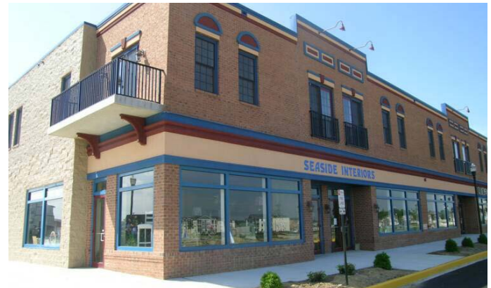
This example shows the use of a recessed entry to identify its location, and changes in material and wall plane to break up the side facade.
