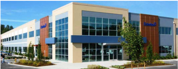
Examples of various techniques in use to break down the apparent mass of a large building, including canopies, recessed decks, recessed top story, and variations in materials and wall plane.
