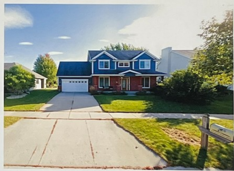
Existing Medium-Density Residential in Swan Creek Neighborhood (5 units/acre)
