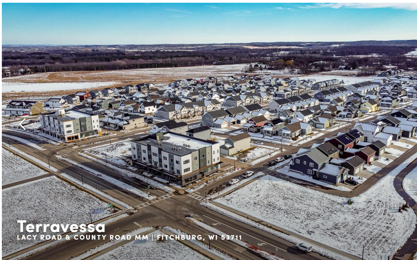
Figure 1 – Terravessa Single-family and Townhomes (T4) looking Southeast. The three-story buildings in the foreground are T5. 3
