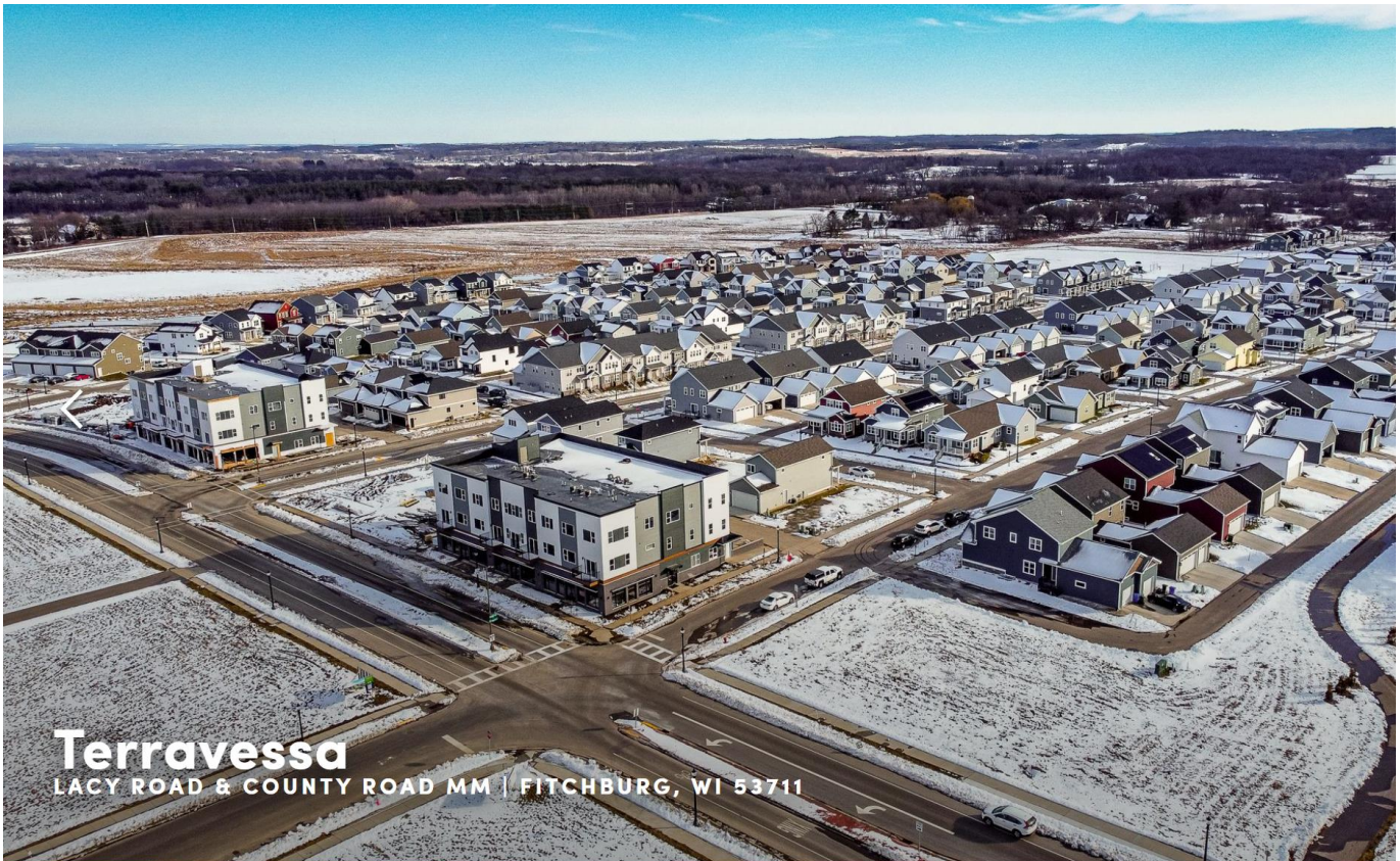
Figure 1 – Terravessa Single-family and Townhomes (T4) looking Southeast. The three-story buildings in the foreground are T5. 3
