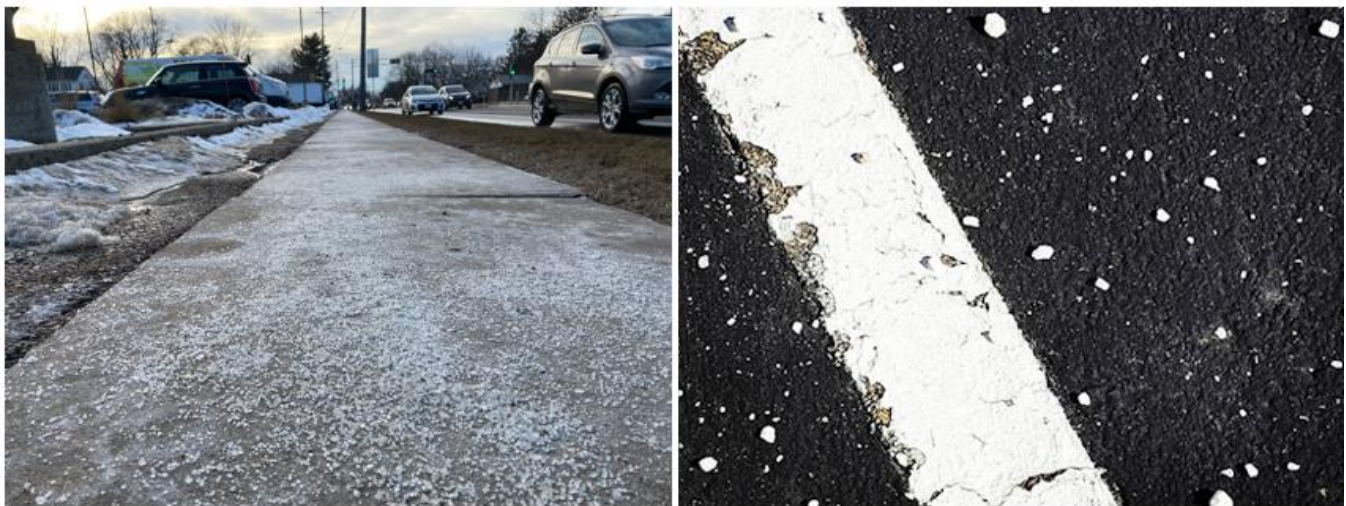
Examples of excessive (left) and proper (right) salt use on concrete and asphalt in the winter.
