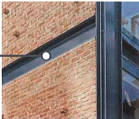
STEEL CHANNEL ABOVE OPENINGS
