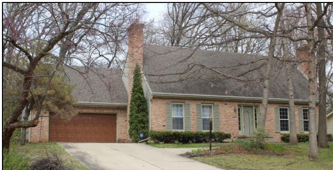
Featured on the 1982 Parade of Homes was this Neo-Colonial Revival style house at 5838 Schumann Drive that was built by the Monson Construction Company for Charles Gietzel.
