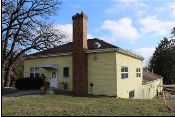
Fish Hatchery office and hatchery itself, built circa 1939, 3911 Fish Hatchery Road.
