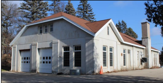
Built in 1940, this WPA-constructed, poured concrete building has historically functioned as a repair shop associated with the Hatchery.
