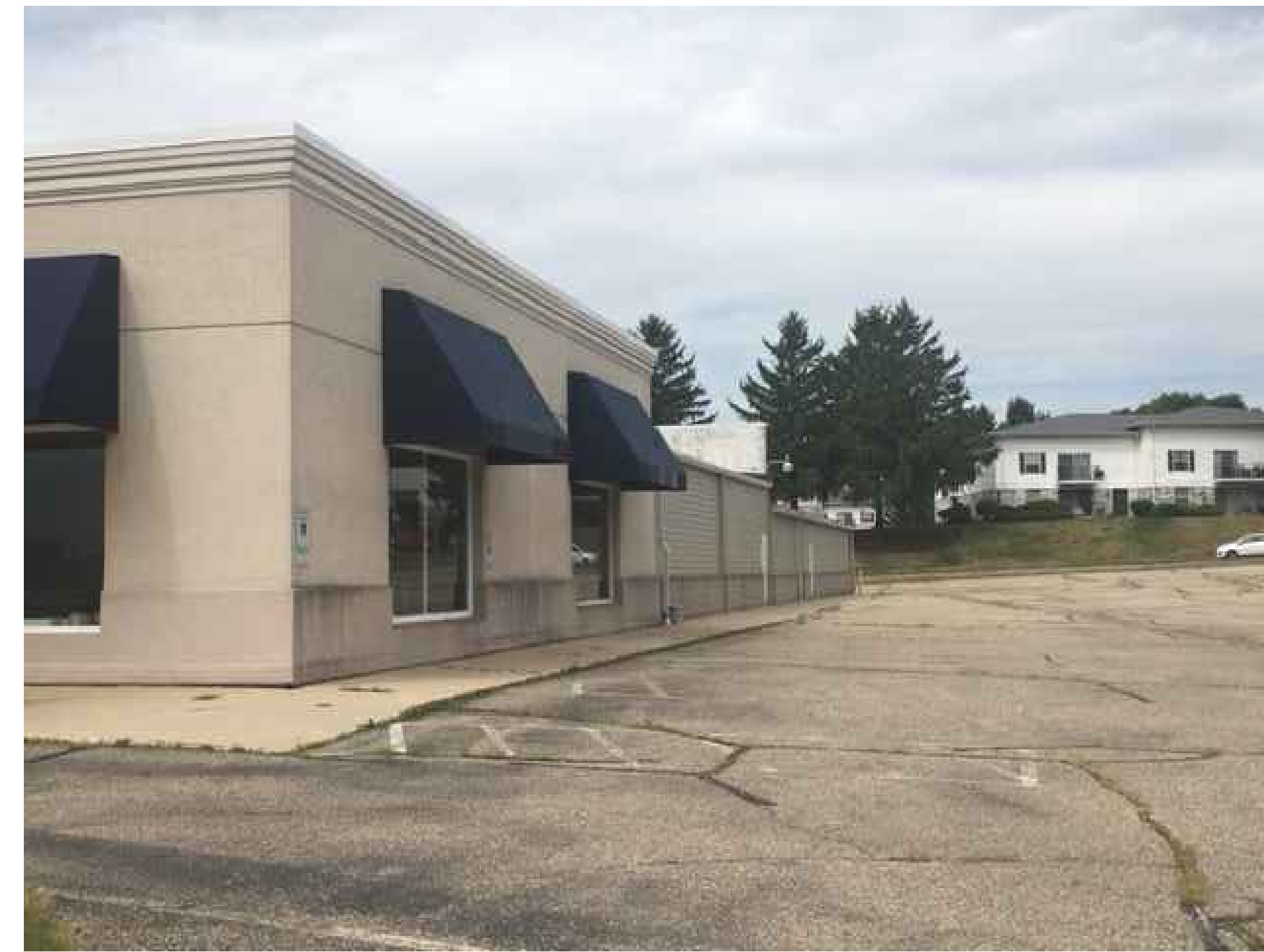
2 Existing North Facade
