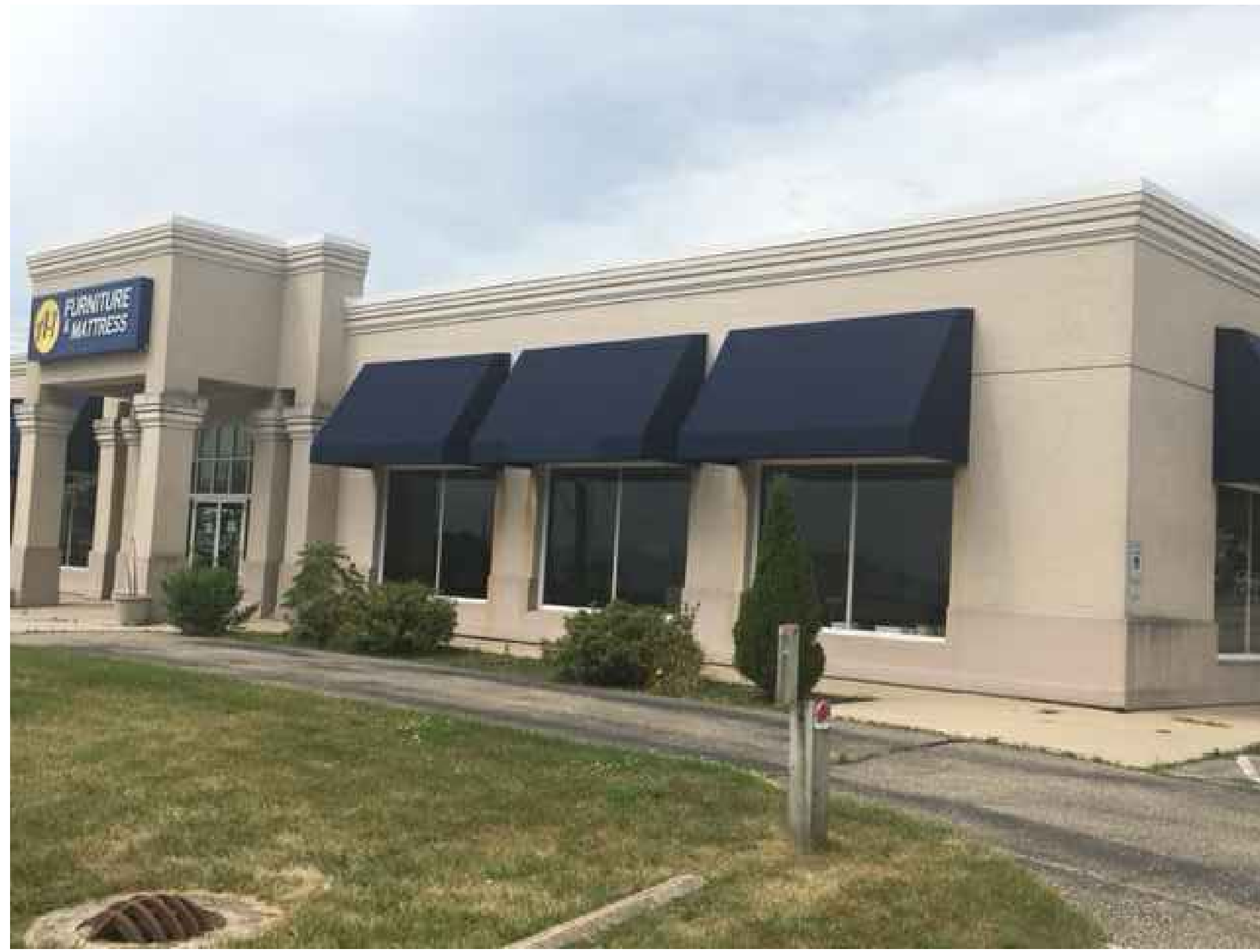
1 Existing East Facade
