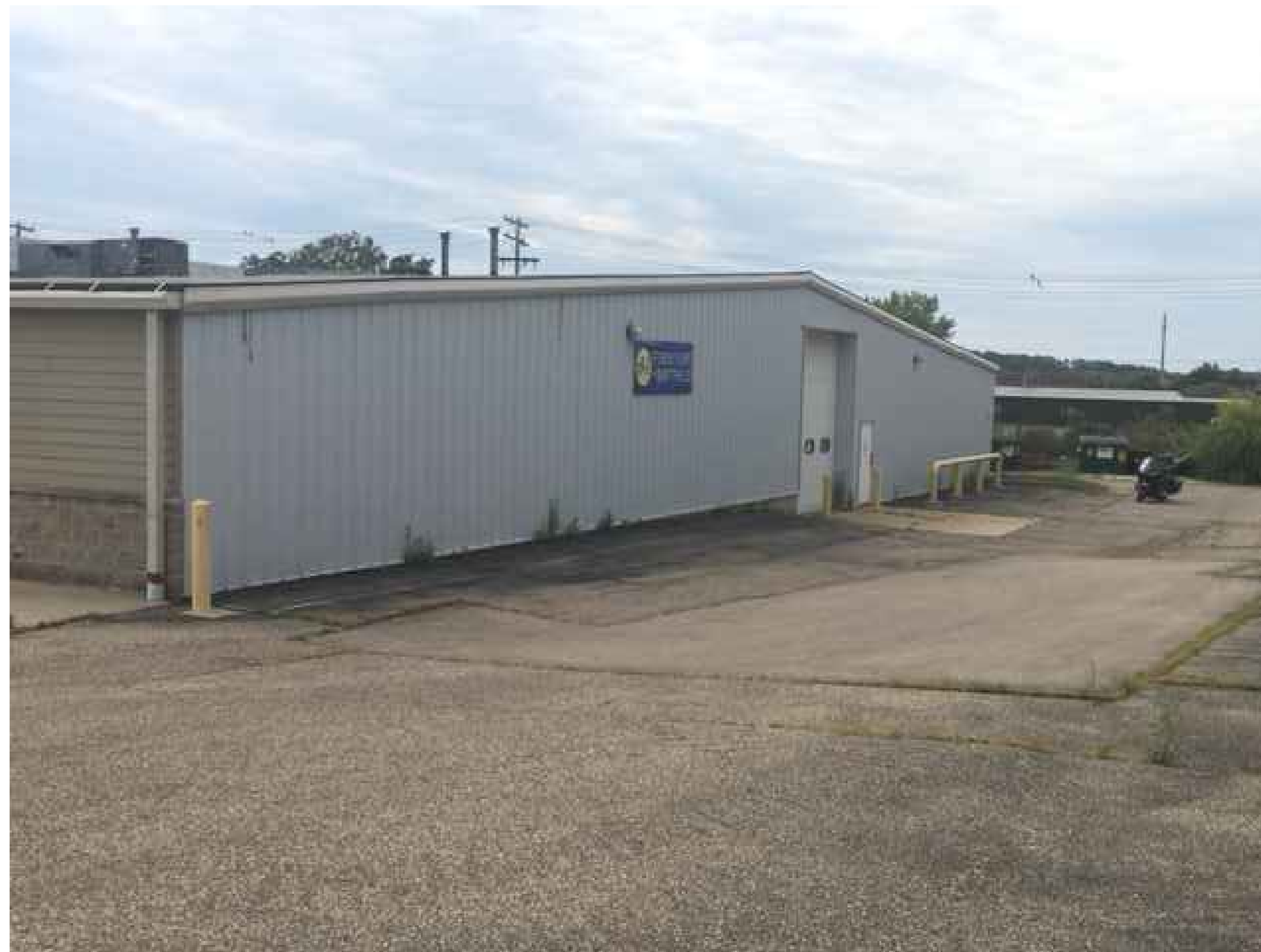
1 Existing West Facade
