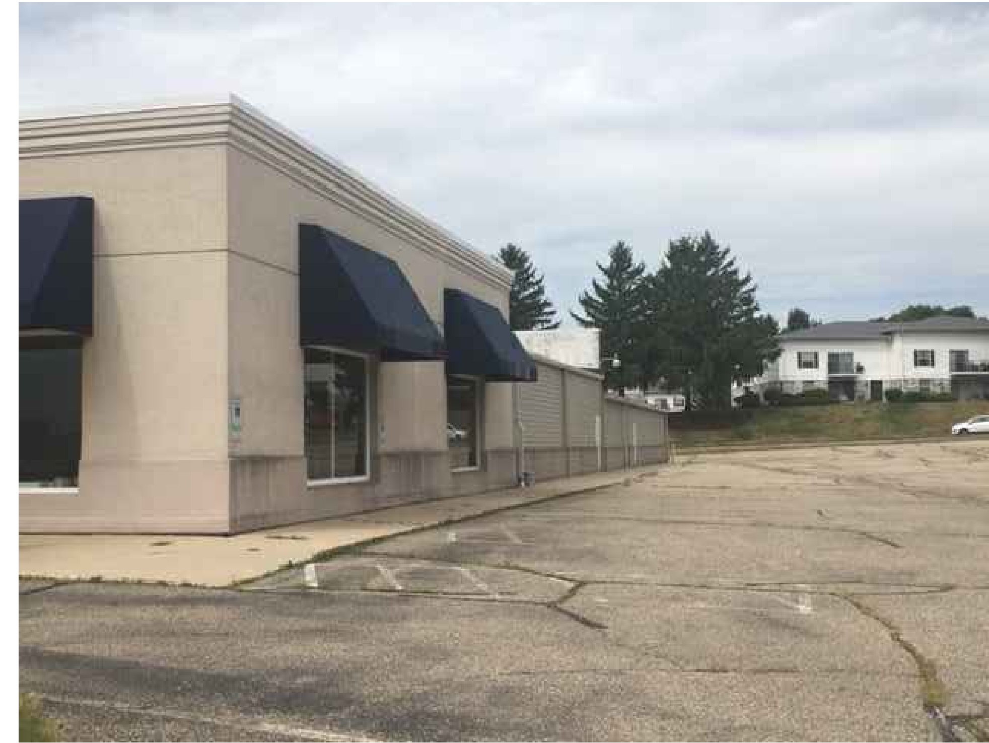
2 Existing North Facade
