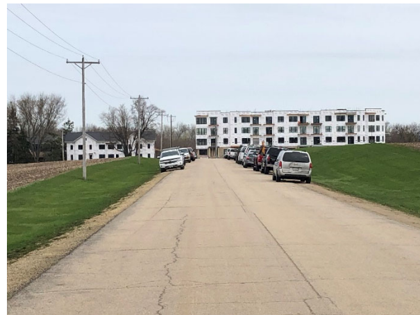
Blaney Road Frontage (view north to The Limerick)
