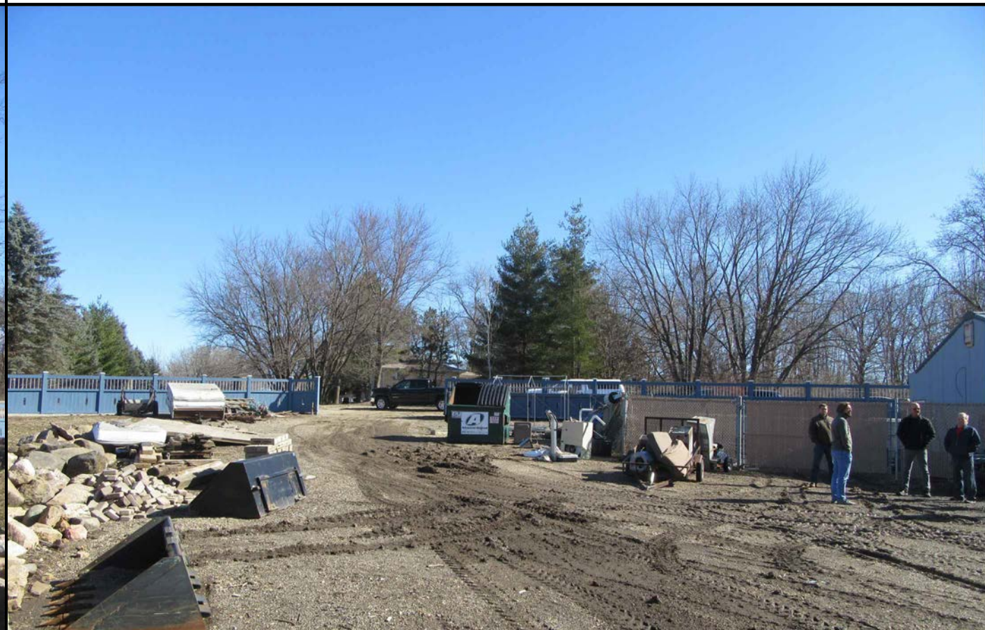
GRAVEL ACCESS DRIVE LOOKING NORTHEAST TOWARDS DELLVUE DRIVE
