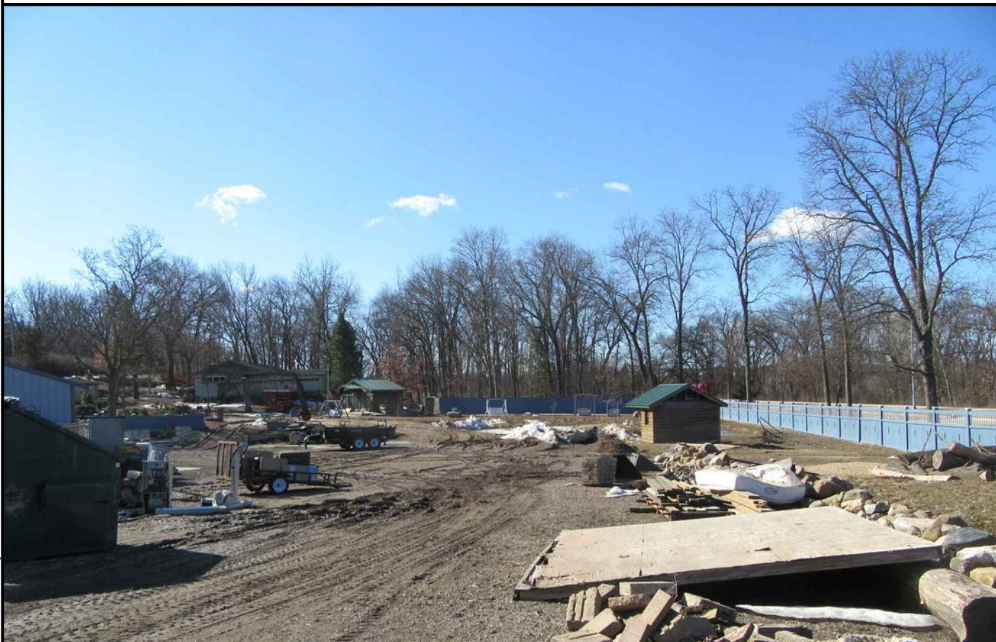
GRAVEL ACCESS DRIVE LOOKING SOUTHWEST
