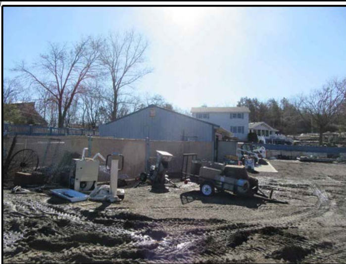
SITE OVERVIEW (LOOKING SE)
