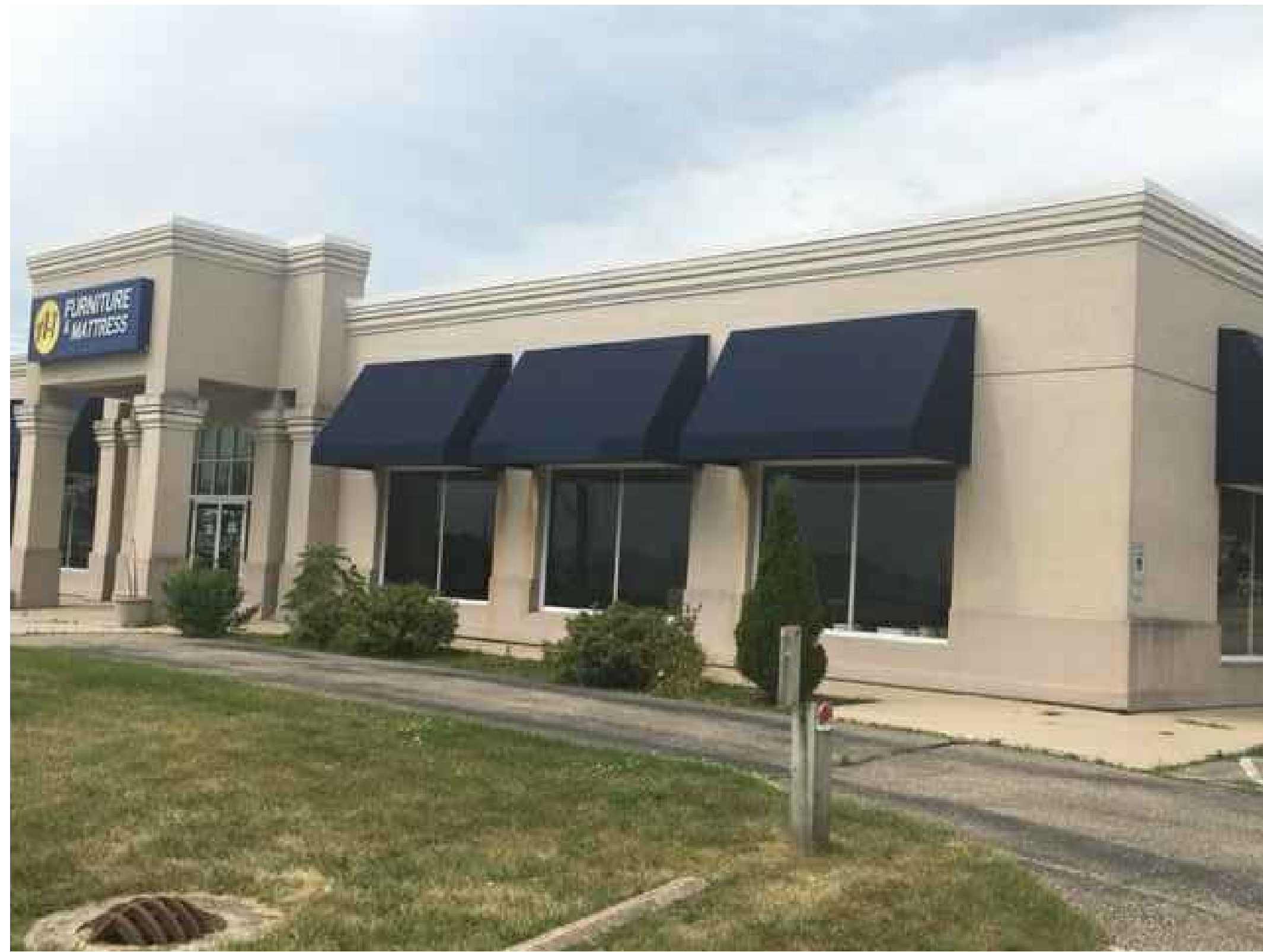
1 Existing East Facade
