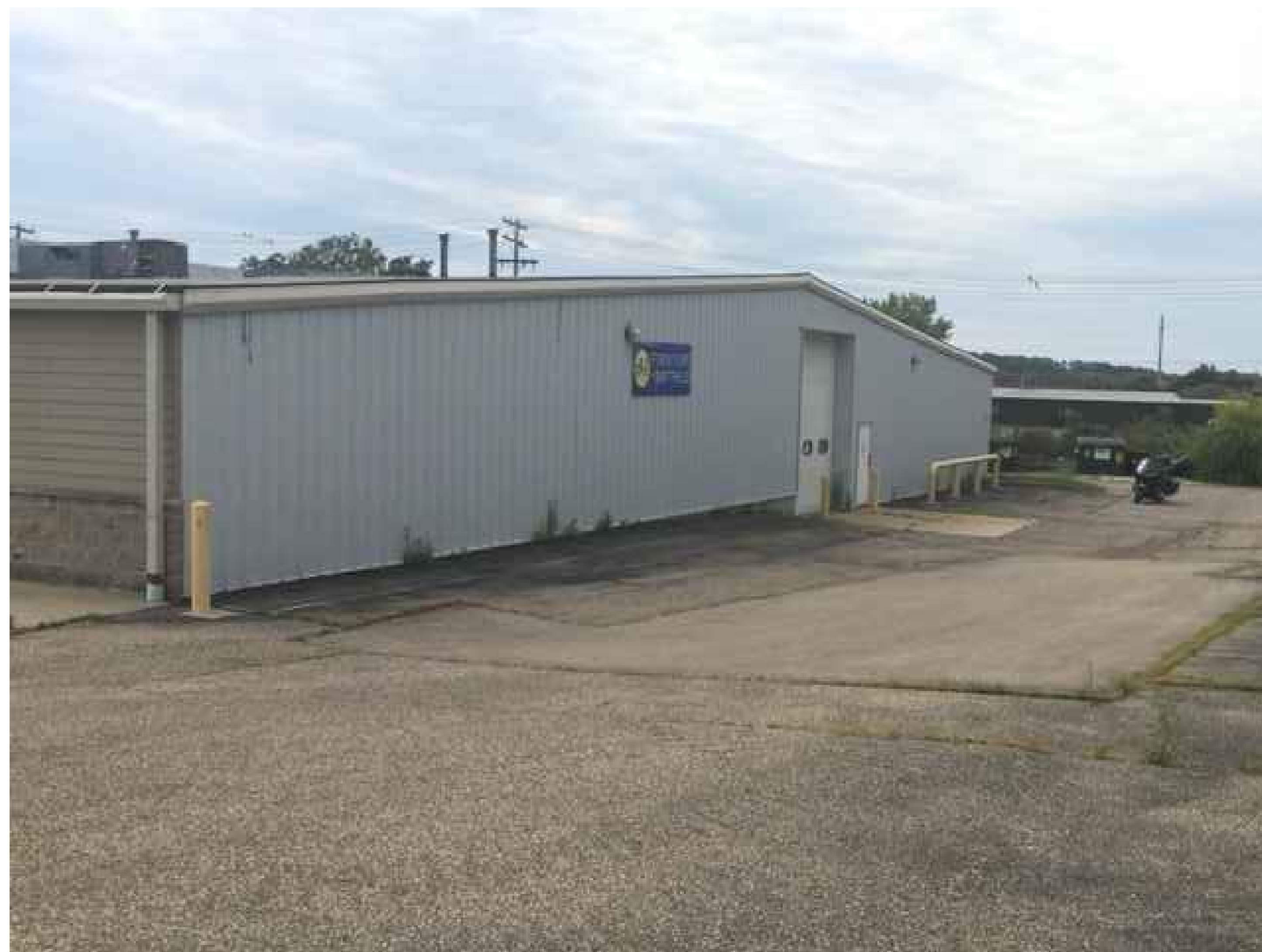
1 Existing West Facade
