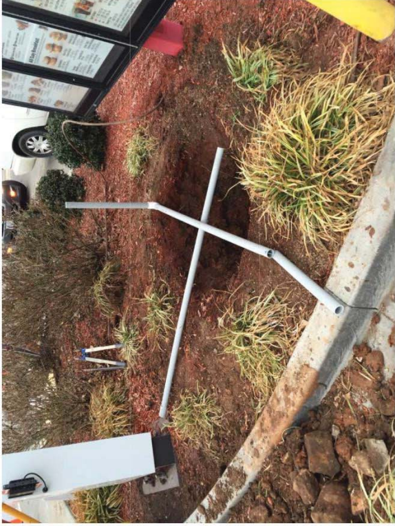
USING JIG TO CONFIRM CENTER OF EXCAVATED FOUNDATION HOLE
