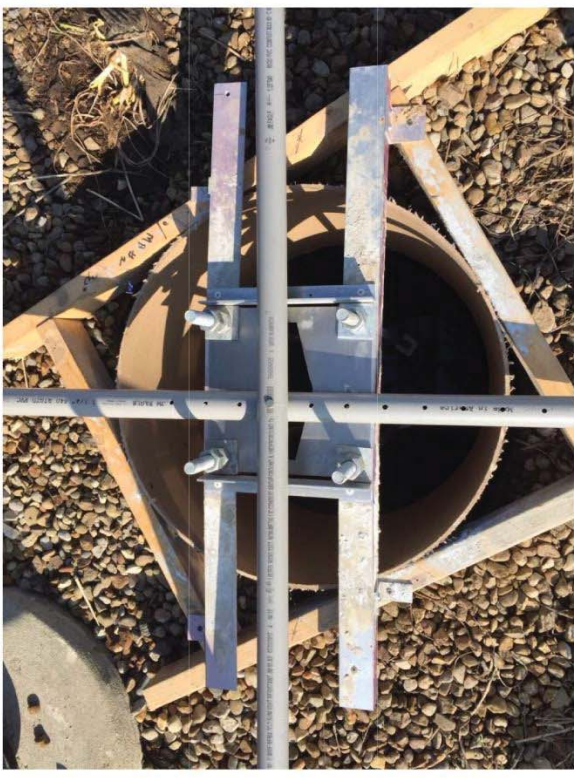
USING JIG TO PROPERLY CENTER AND ALIGN ANCHOR BOLTS
