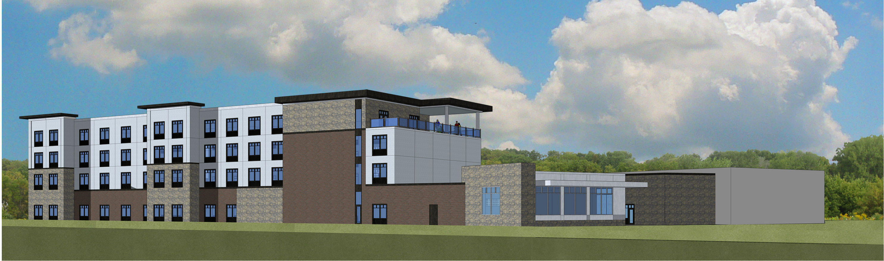
view from Fish Hatchery Rd. to NW
