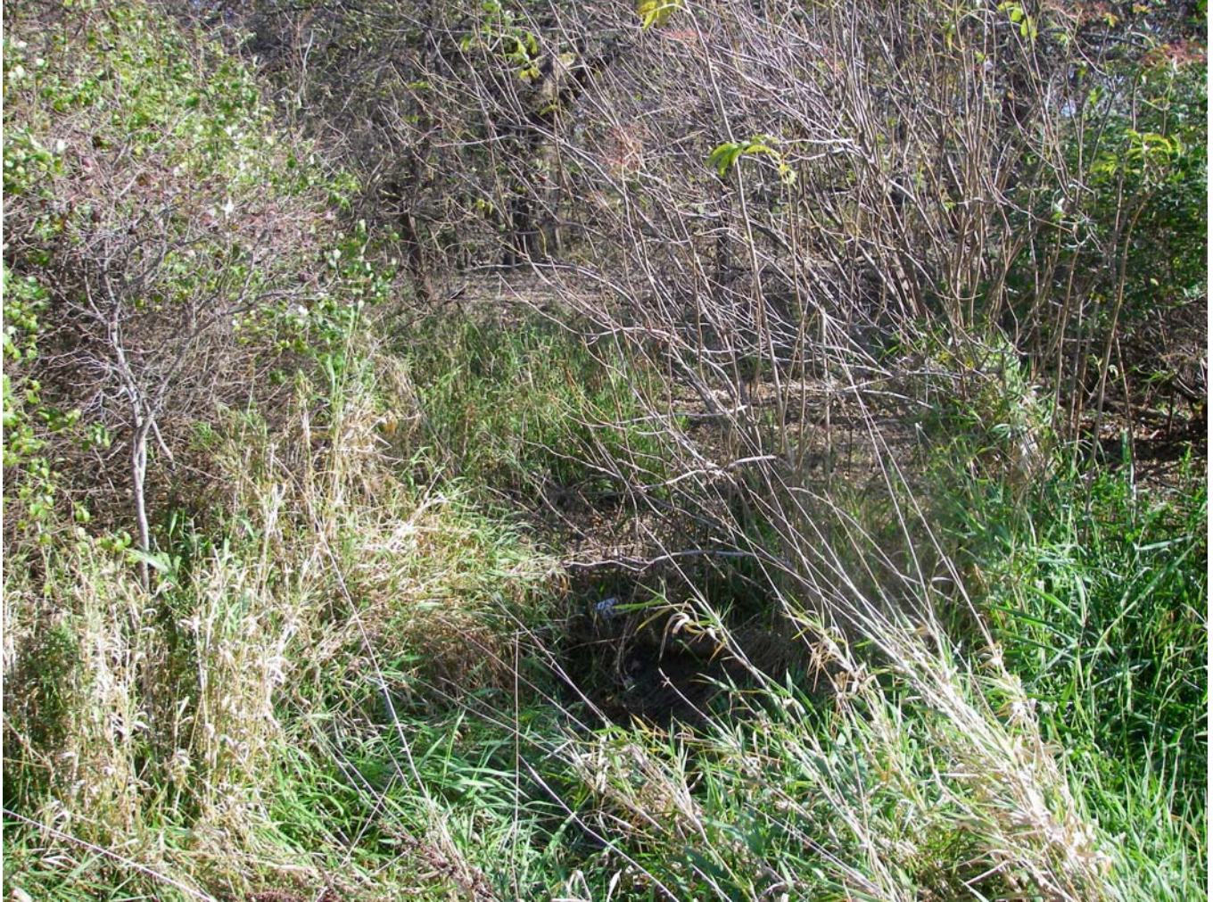
Photo 07. Discharge Point of W-3.JPG
