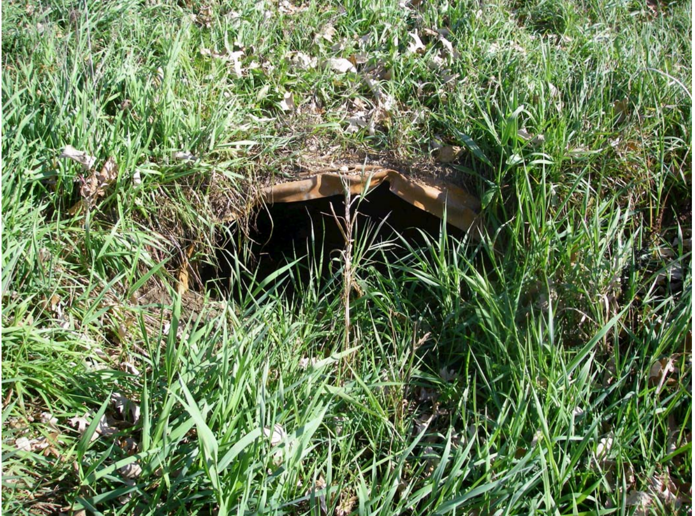
Photo 01. Culvert at W-3.JPG
