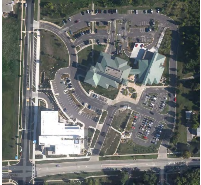
Civic Center Campus Aerial View
